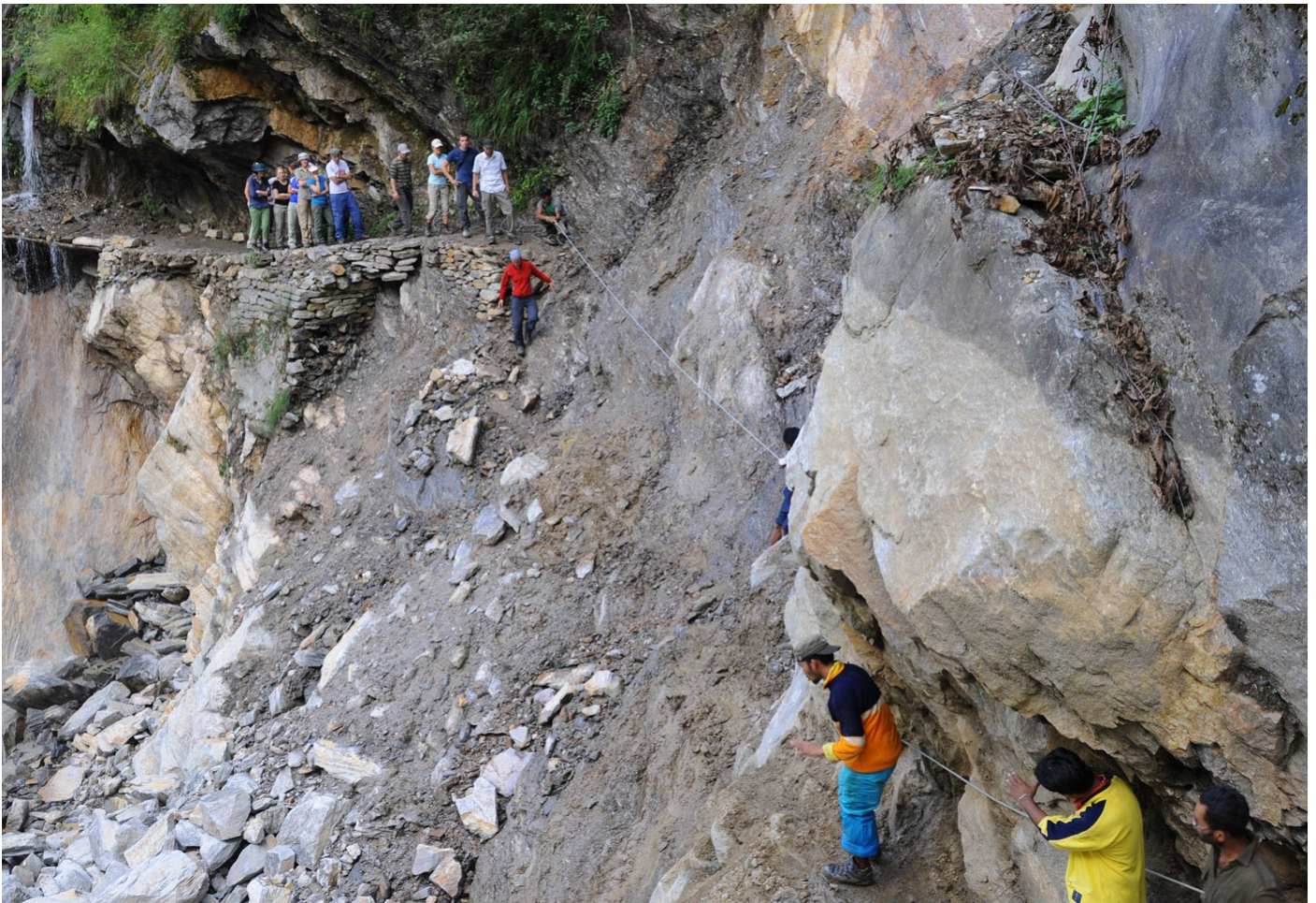
Bridging the gap: landslide in the Gori Valley.
